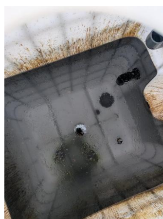
Figure B - Extracted coal tar collecting in bunded containers at the surface before being disposed of to a suitably licenced facility.
